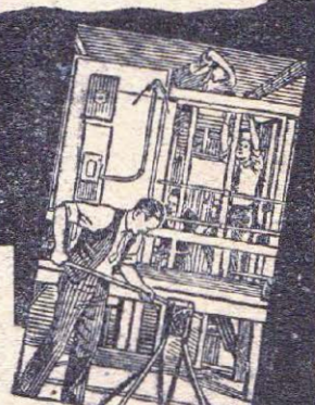
HOUSE WIRING only one of the many branches you "Learn By Doing."
